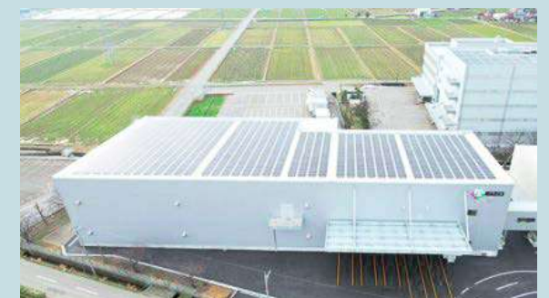
EIZO Corporation Logistics Building (Japan, FY2022)
