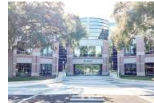
EIZO Rugged Solutions Inc. acquired a new building. (Photo taken in 2022)
